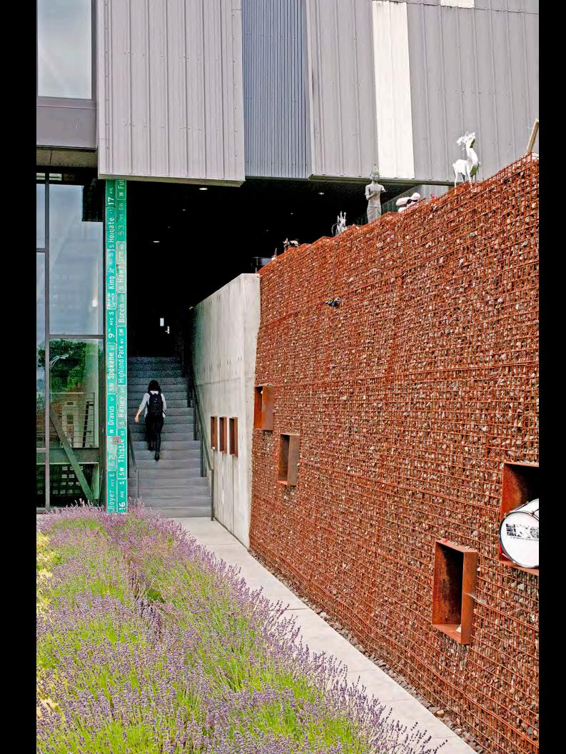
The site design includes over 600 linear feet of custom gabion veneer walls. Their highly textured presence are designed at a scale to draw interest from vehicles on adjacent roadways and from pedestrians on the site.
